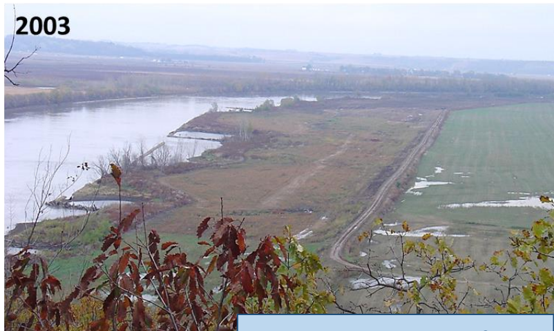
Levee construction on accreted land
